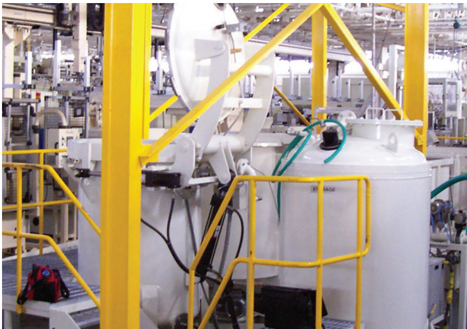
Automatic Installation at Suzuki Powertrain
